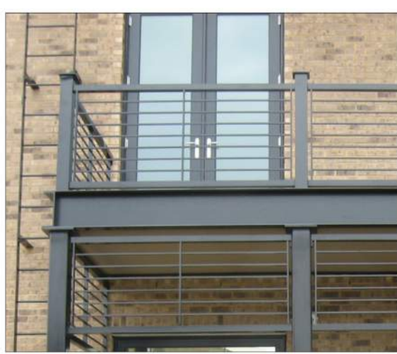
① STEEL BALCONY / RAILING
