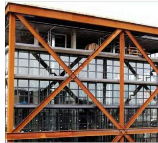
9 STRUCTURAL STEEL FRAME
